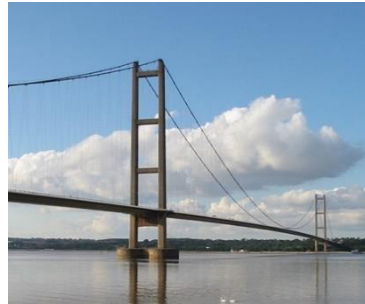
The Humber Bridge
